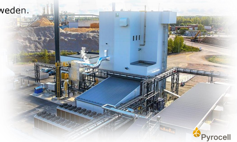
Pyrocell fast pyrolysis plant (25 MW th ) in Sweden
